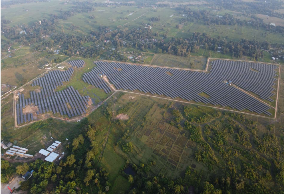
Installation of 29 MW Solar power plant.
